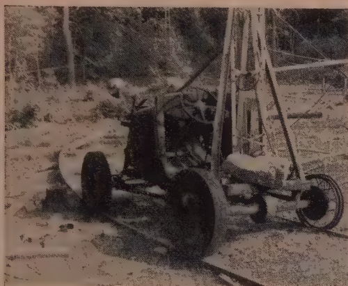
Truck on guide rails.
