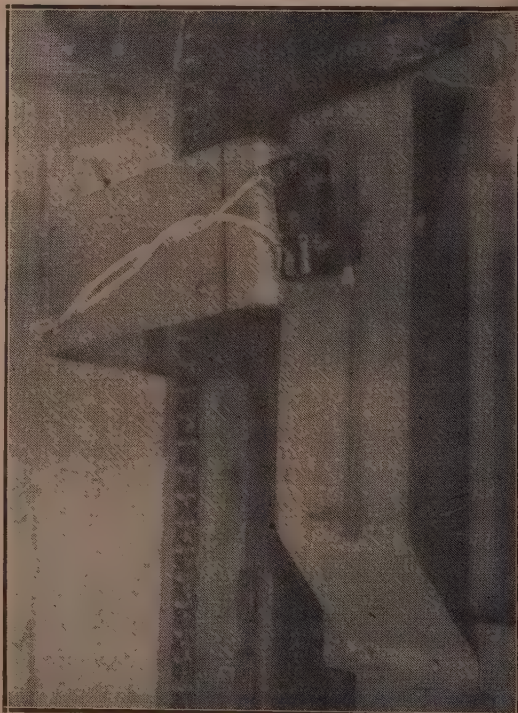
Fig. 3. Detail of the "slide" attached to the garage door to engage the microswitches and which act as "limit" controls.
