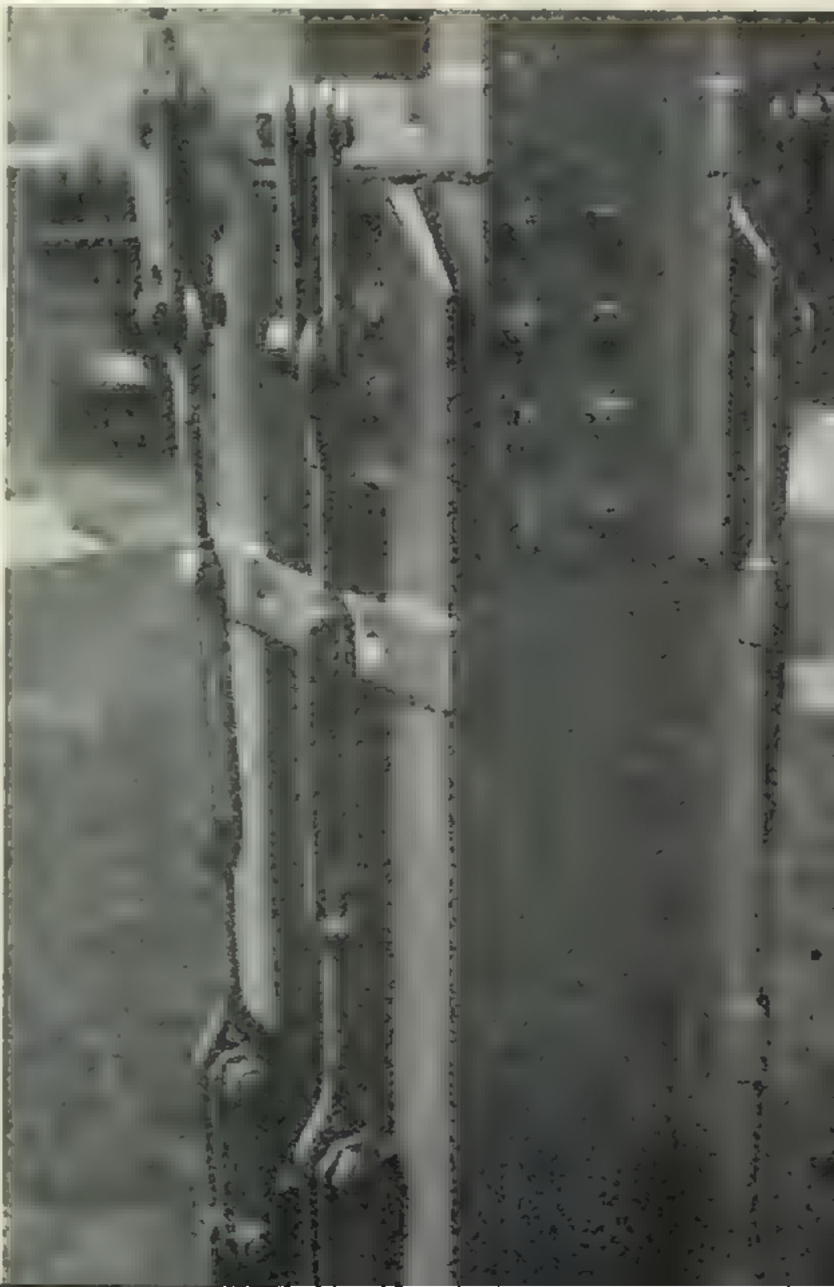
(Below) Detail of the outrigger lower terminal and the joining of the base and first sections
